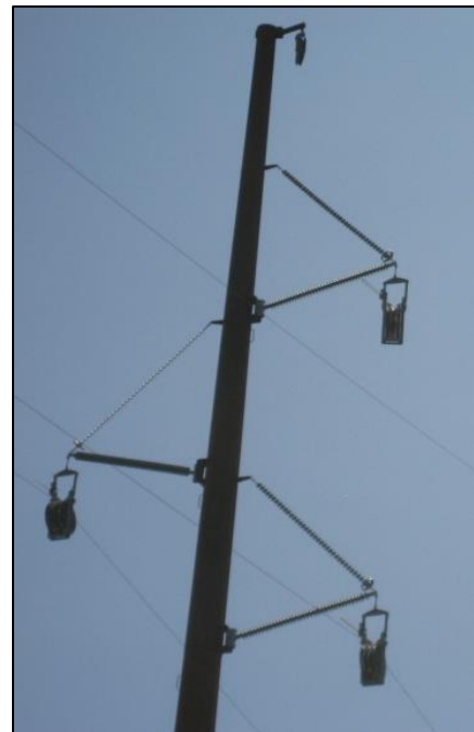
Fig. 1 – Stringing of Braced Post
