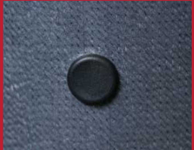
FIG. 10.2. Hole plug installed
