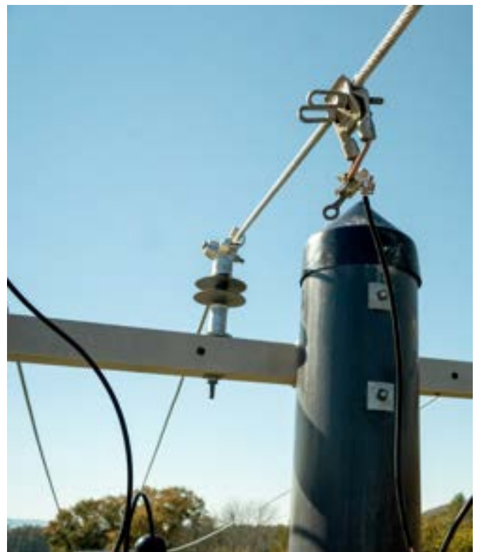
FIG. 8.4. Crossarm connection with other distribution products
