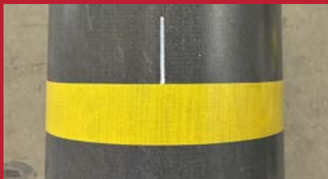
FIG. 7.1. Groundline marking - yellow tape
