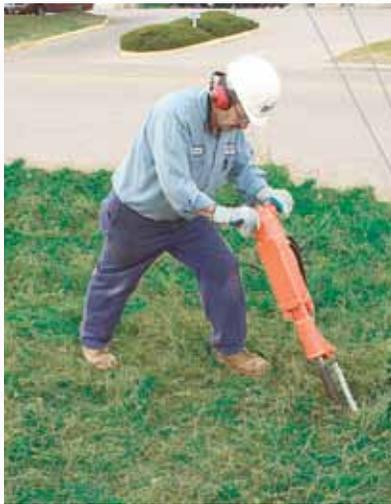
② Drive the anchor to the proper depth, adding sections of drive steel as needed.
