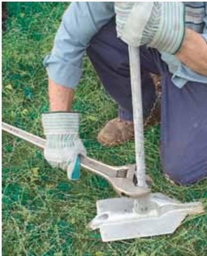
① Thread a standard power hub anchor rod into the threaded shackle of the Manta Ray Anchor.
